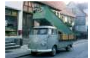
"Transportable" Lauber wood dryer in the past (1968).
